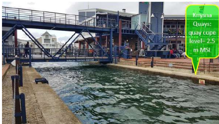
Figure Aa.1-2: Photograph (courtesy Nichelle Swanepoel) of Knysna Quays Marina during high tide (approx. 16:00) on 28 October 2019. Cope level of the quay walls are at +2.5 m above sea level
