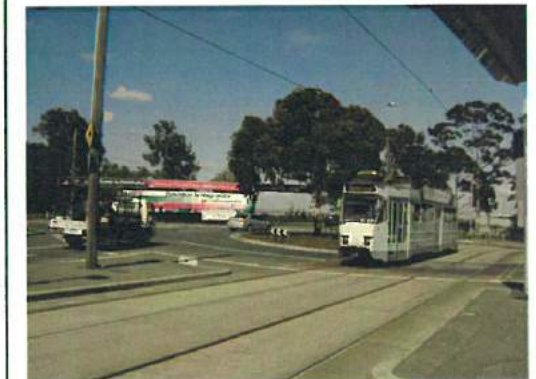
Photo 5.8.1.2 Tram stop at Flemington Racecourse, Australia (source: www.crudeoil_peak.info )
