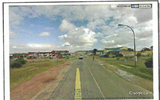
Photo 5.6.1(a) Dana Bay gateway node showing disjointed collection of commercial buildings and little attempt at any civic design and landscaping (source: Google Earth, 2017)
