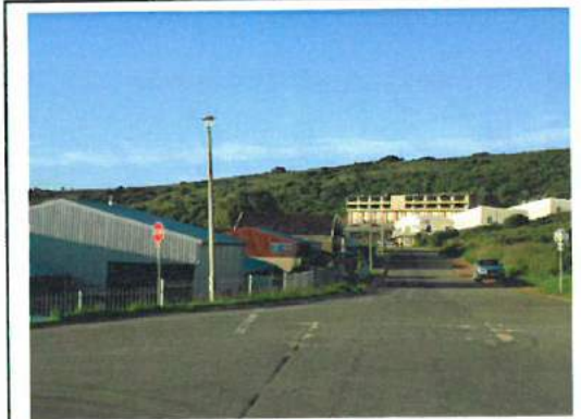
Photo 5.9.2(d) Image showing variation in urban character, with residential and industrial buildings across each other (source: CNaV Africa, 2017)
